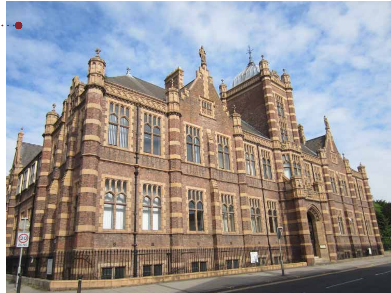
Old Technical Building G.G. Hoskins 1894-97.
