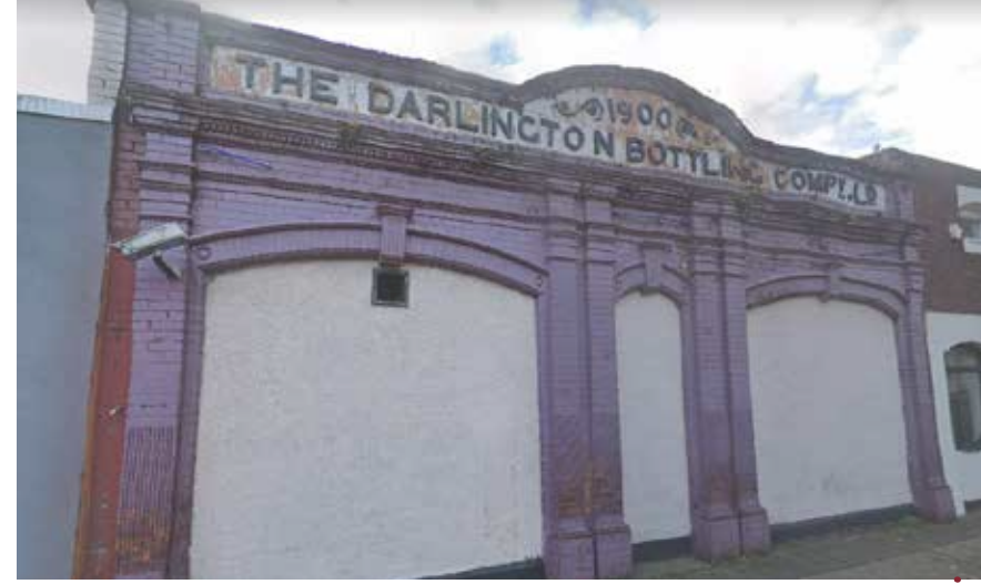
Existing Darlington bottling company arches to be retained to create new pedestrian access.
