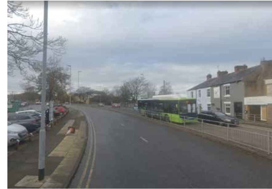
4. View down St Augustine's Way with the site visible on the right.
