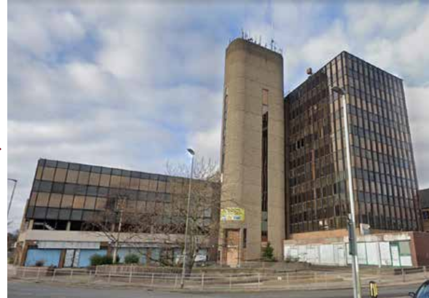
3. View back from northgate roundabout towards northgate house office
