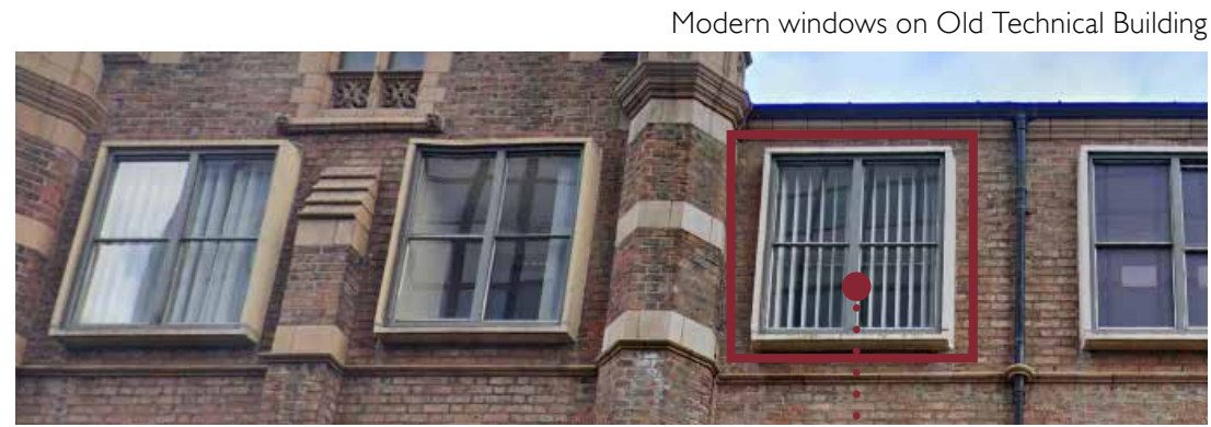
Modern windows on Old Technical Building
