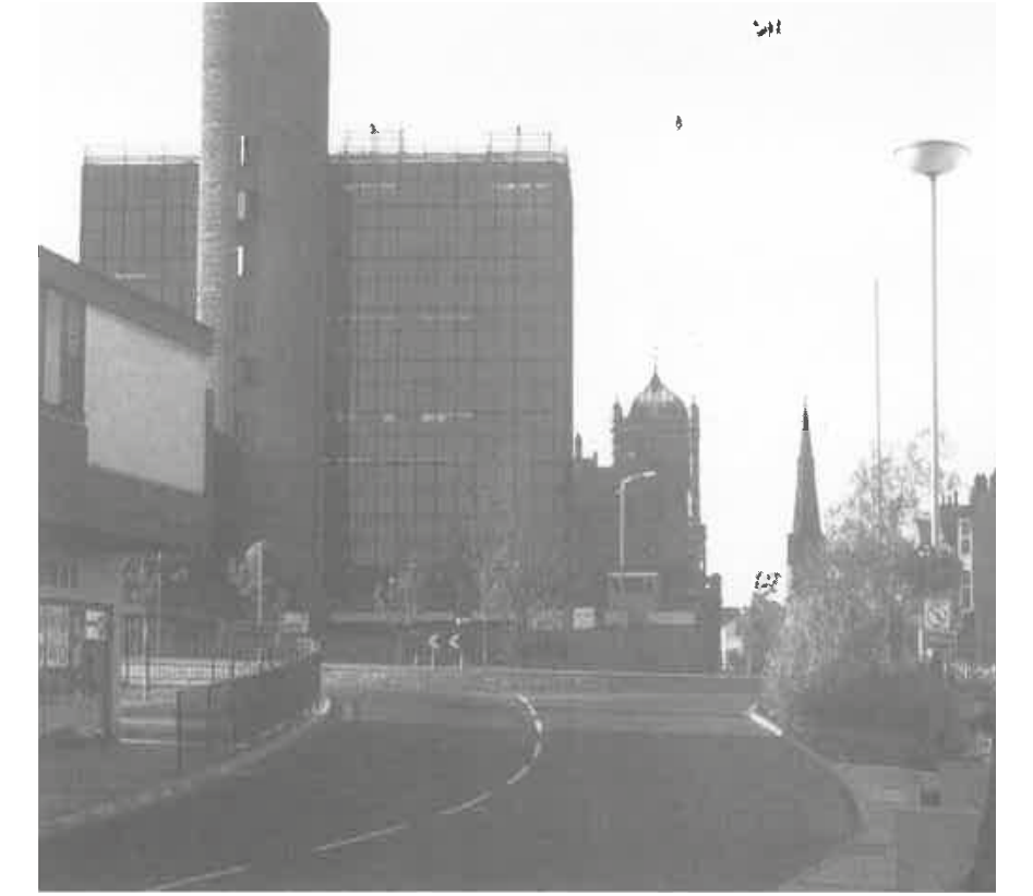
Northgate house completed in 1977
