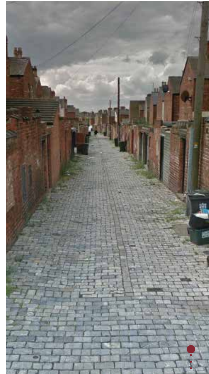
Blue 'Scoriae' bricks laid in nearby alleyways.
